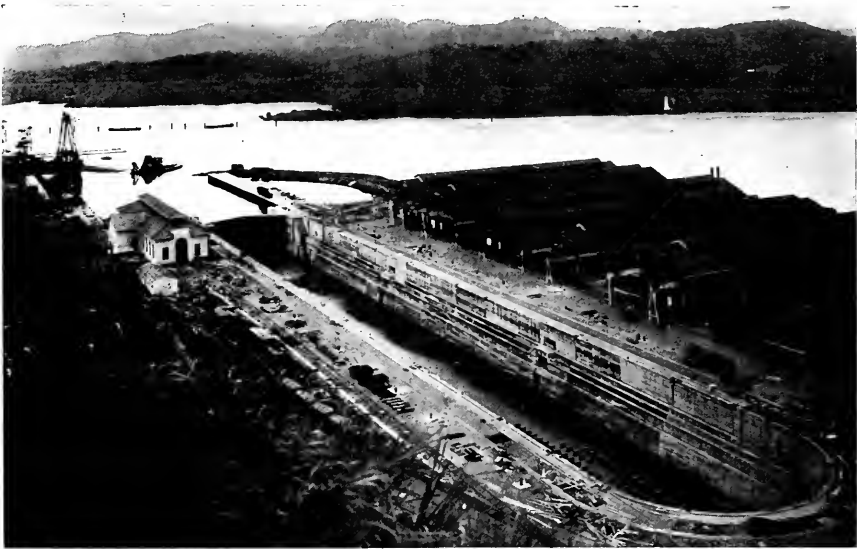
General view of new 1,000 foot dry dock at Balboa, with coaling plant on the left and shops on the right. A dredge is shown cutting a channel through the earth cofferdam which protected the dry dock entrance during construction. The canal channel lies between the shops and the light tower shown on the opposite bank. Ships coming from the Pacific move across the picture to the right. At the right of the shops as shown is a new group of piers.
